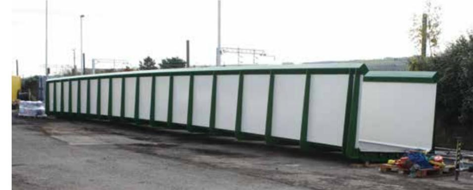
**ACCESS FOR ALL BRIDGE FOR DUNBAR: A new footbridge was lifted into place by crane (below) and lifts were installed as part of a £13 million scheme at the East Coast main line station at Dunbar, together with a second (new) northbound platform to accommodate a 10-car train**
