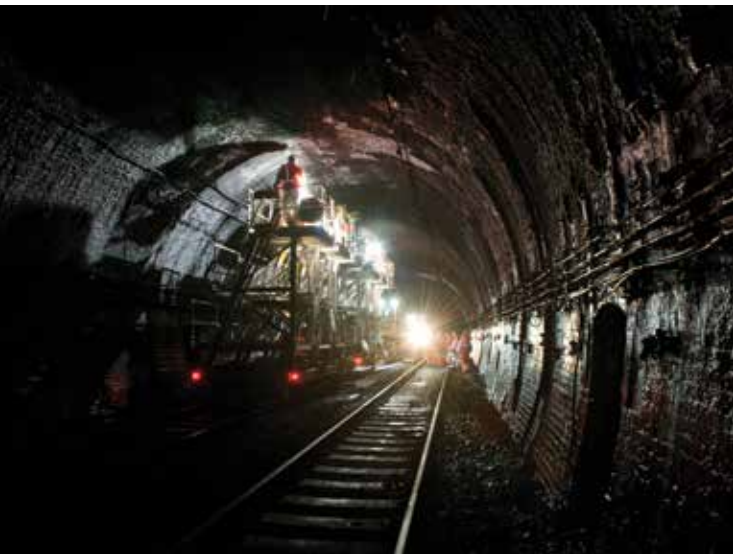
JOB WELL DONE: Severn Tunnel was closed for six weeks up to 22 October for electrification equipment to be installed
