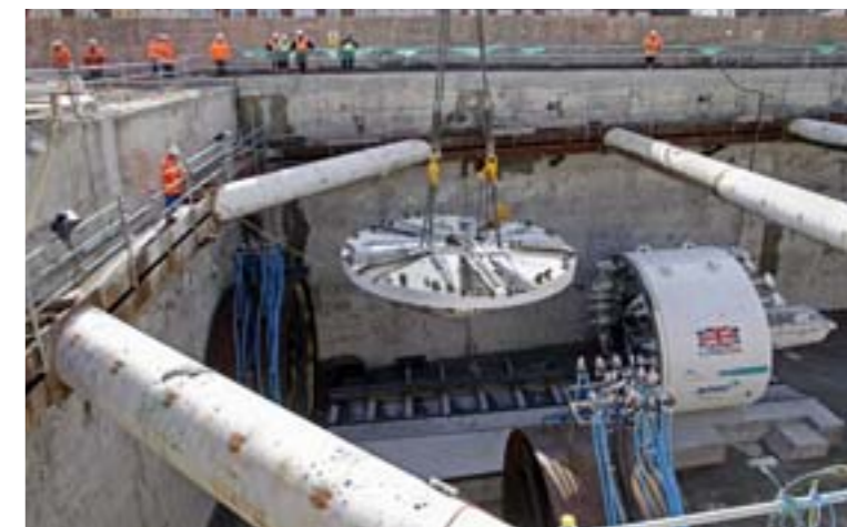
DOWN IT GOES: The boring machine is craned in Picture: DLR
