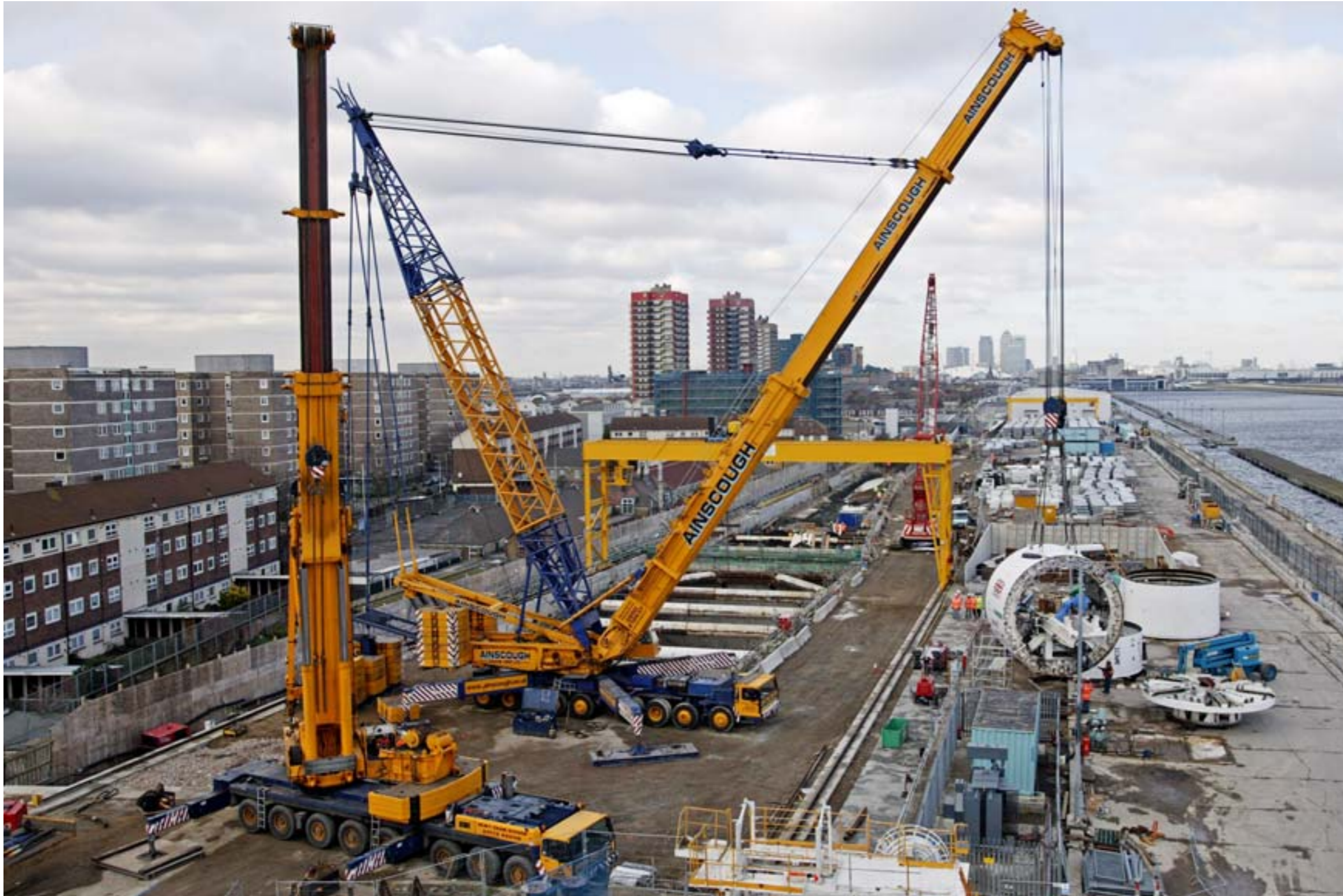
WAY TO GO: Cranes beside King George V dock lift the boring machine before lowering it into the trench for the new light rail line from north of the river to Woolwich Picture: DLR
