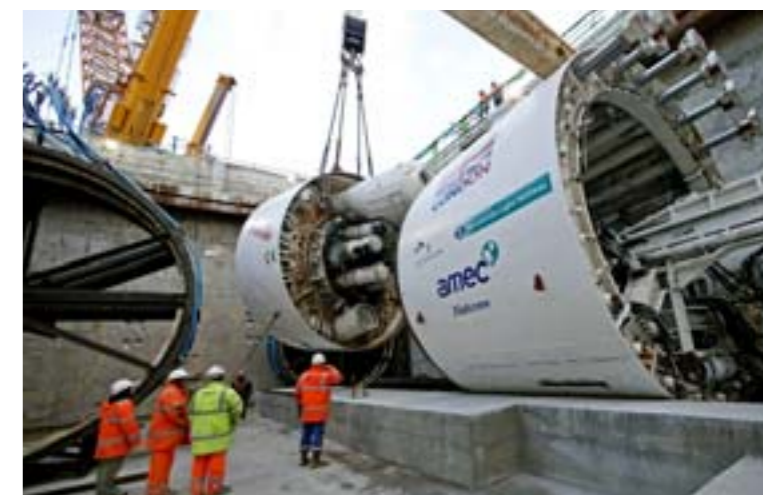
ALL SET: The 540-ton boring machine is assembled Picture: DLR
