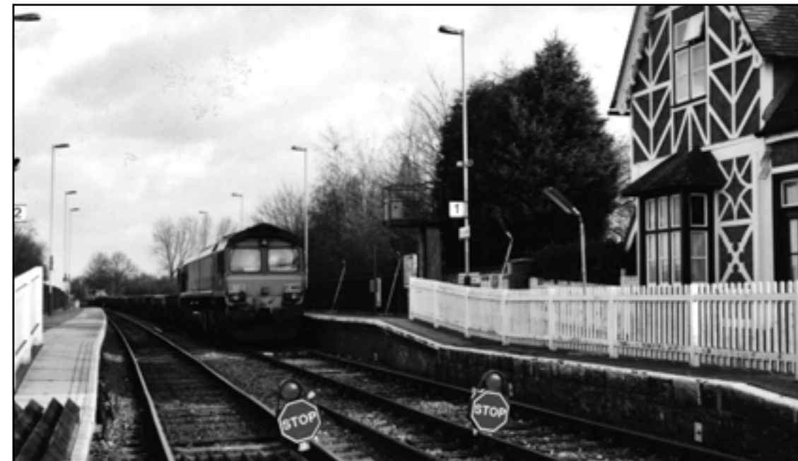
A works train at Millbrook station. See letter headed Modernisation
