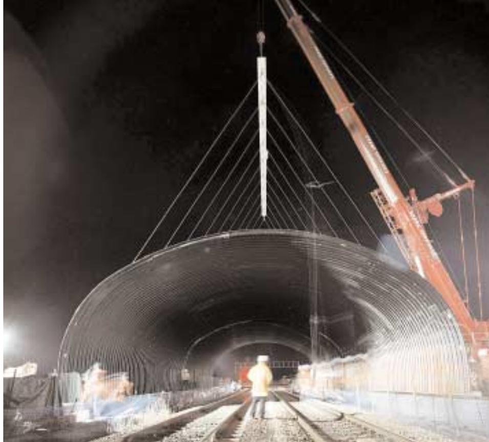
*In a move that contractors believe will transform the way road and railway links are constructed in the UK, the first-ever corrugated steel tunnel arch support has been installed for Stockton-on-Tees borough council.*
