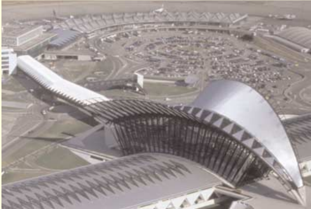
Lyon Saint Exupery station. The roof was designed to look like the wings of a bird taking off
