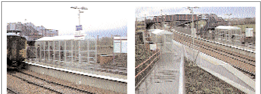
The first station to open in the 21st century: Dunfermline Queen Margaret station began operation in January and is well situated for the hospital, which has parking problems like many other hospitals. The next station to open in Fife should be in east Kirkcaldy. This will complete the long gestation of stations in south Fife that started with Thornton. Congratulations to Fife Council for progressing these despite endless problems.
