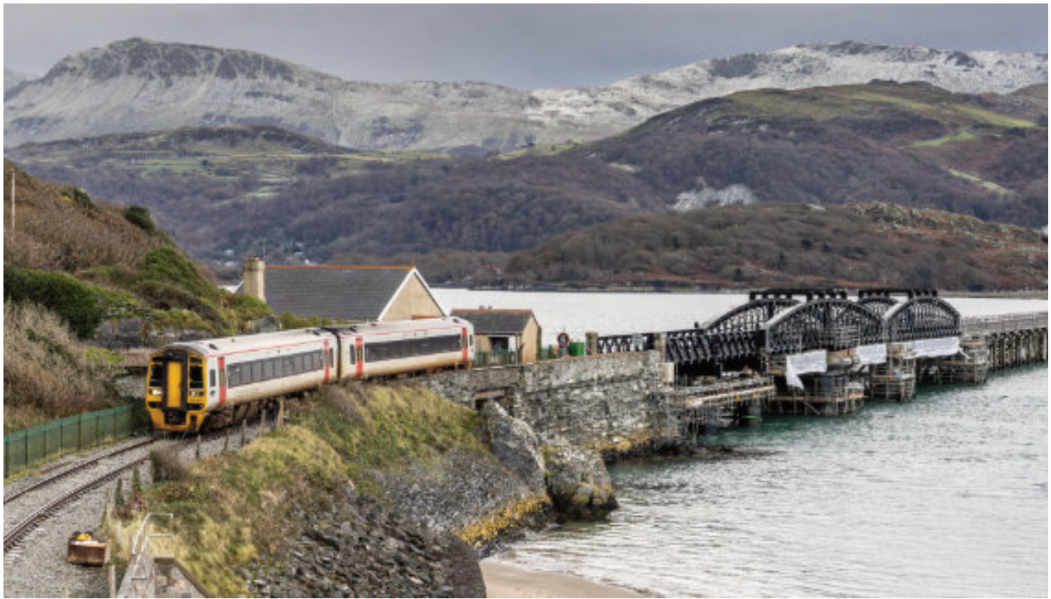
BACK IN ACTION: Pont Abermaw (Barmouth bridge) has been renovated after a major £30 million upgrade. The rail service was suspended for three months in autumn 2023 but resumed in December. Network Rail's picture shows a Machynlleth to Pwllheli train, Afon Mawddach and snow-covered Cadair Idris in the background
