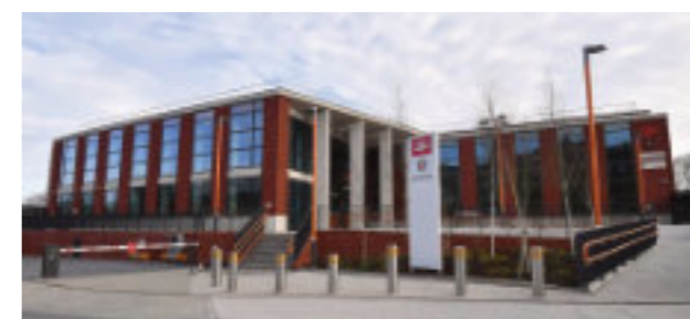
UNIVERSITY STATION Photo West Midlands Rail Executive
