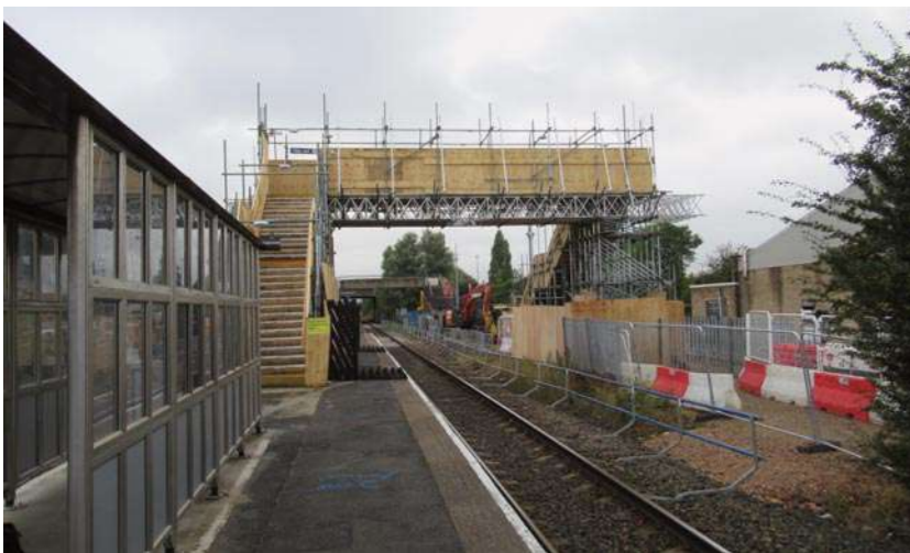
BILLINGHAM STATION: Looking south towards Stockton and Middlesbrough with one new footbridge in place.
