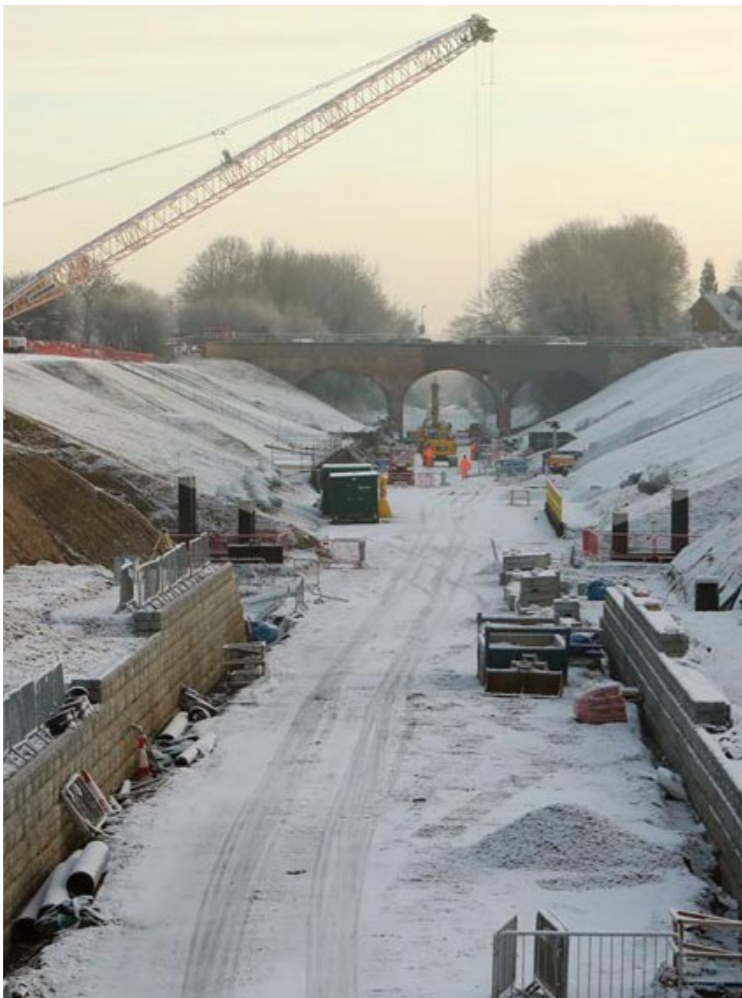
FROZEN HEART: Platforms were being constructed as snow fell in December last year at Winslow station which will be at the heart of East West Rail when it transforms travel between Oxford, Milton Keynes and, eventually, Cambridge. More than 500 pre-cast concrete platform units were lifted into position using a crane with a boom longer than Nelson’s Column
