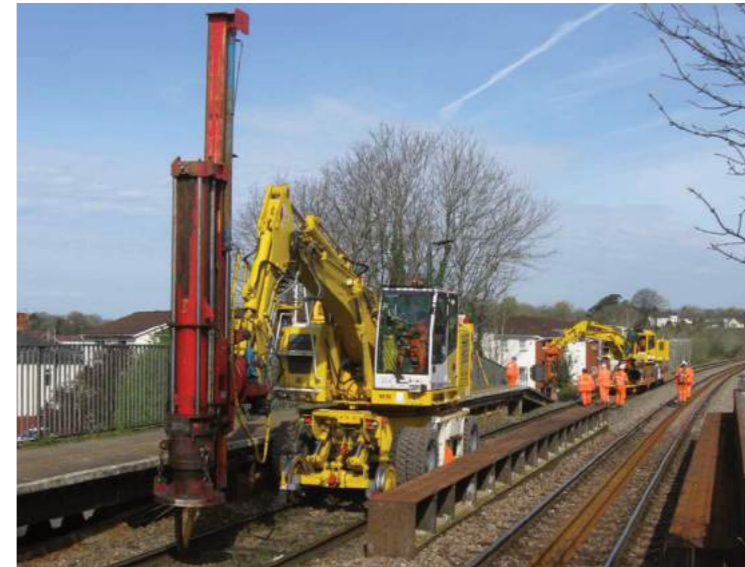
Two machines for driving piles into the ground working at Waun-Gron Park station on the Cardiff City line in April, part of the work to electrify the core valleys lines
