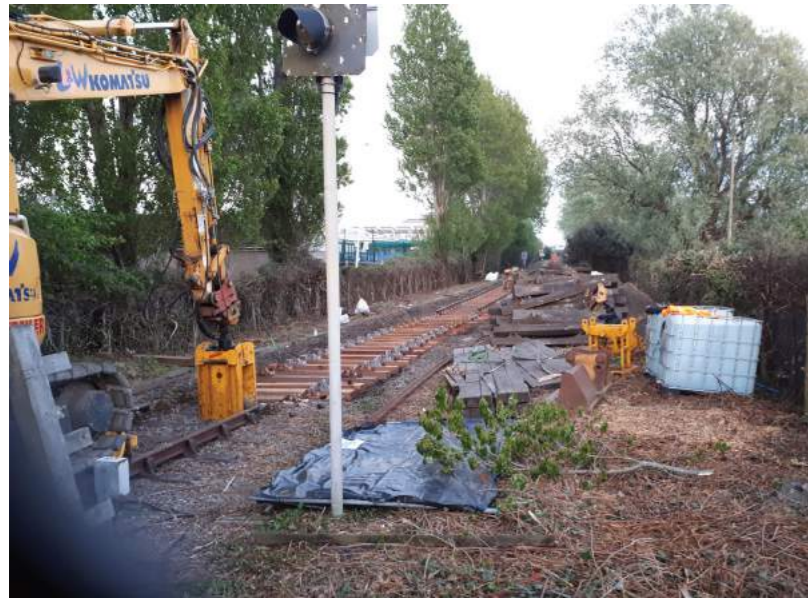
FIT FOR FREIGHT: The Hamworthy branch gets new sleepers in April
