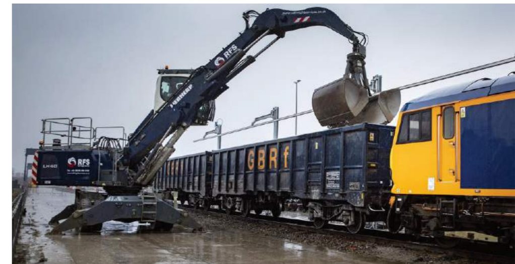
MOVEABLE: The 25kv power supply is retracted to allow cranes space to load trains
