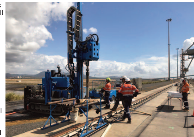
LEVENMOUTH: Sonic drilling under way before reopening
