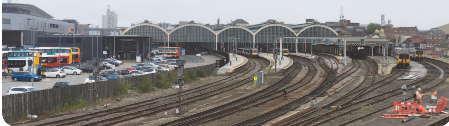
HULL PARAGON STATION: Open access operator Hull Trains provides direct trains to London King's Cross from here
