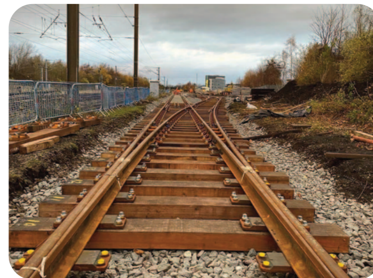
DARLINGTON: Relaid siding for 750 metre long freight trains
