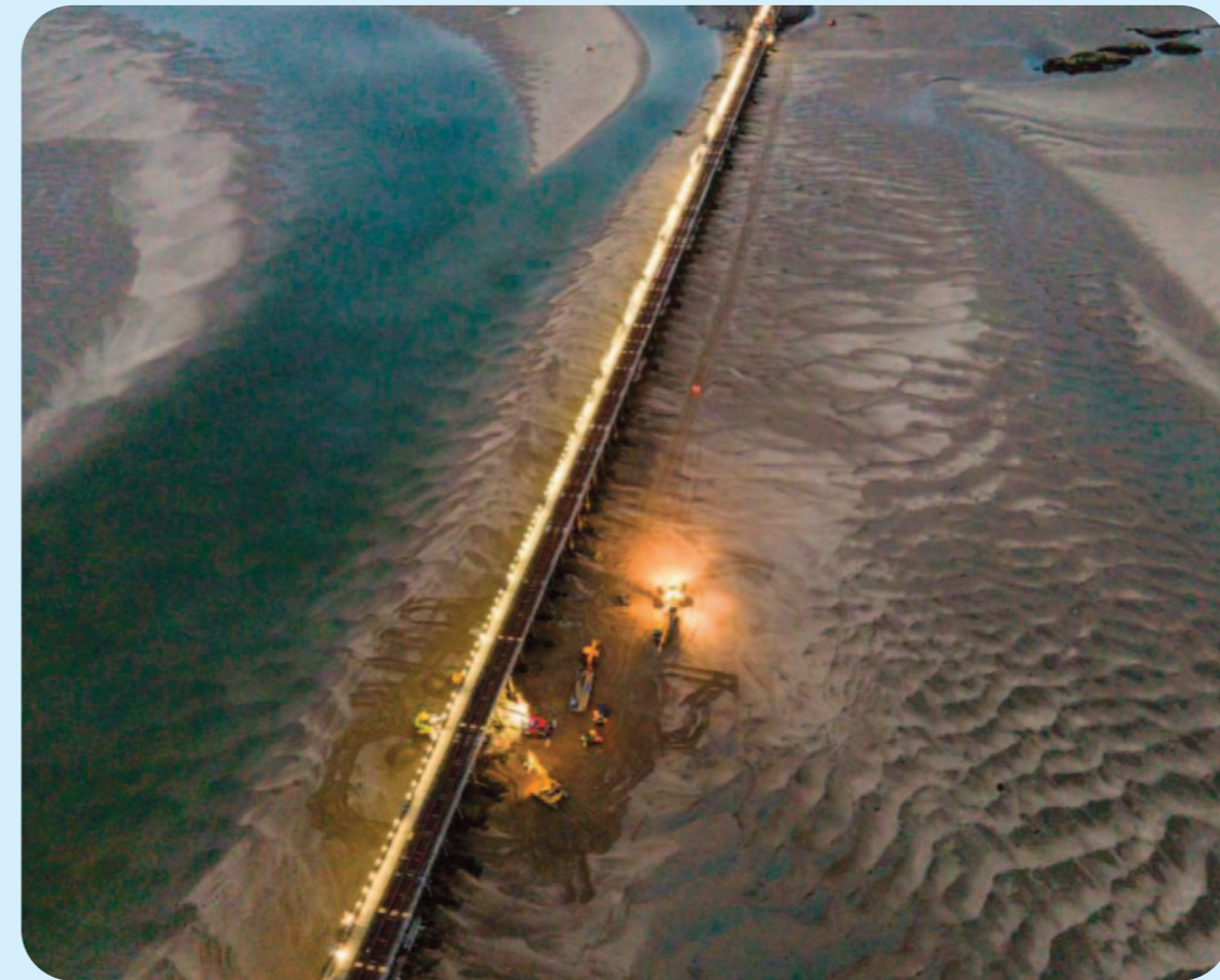
BARMOUTH BRIDGE: This half-mile vital railway over the Afon Mawddach estuary is currently being repaired by Network Rail in a £25 million project. Rail-mounted cranes are supplemented by caterpillar-tracked vehicles at low tide. The strong currents can be seen in the megaripples near the bridge. Barmouth Bridge survived the Beeching axe and the 1980s shipworm crisis
