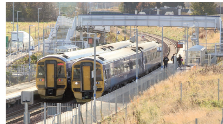
SHAWFAIR: It now claims to be the best connected new town in Scotland – thanks to the opening of the Borders Railway
