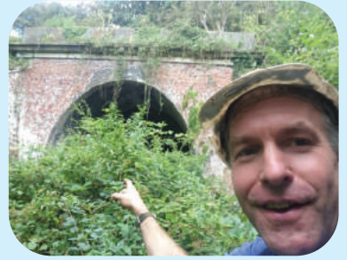
Welland Rail's Owen O'Neill at Morcott Tunnel which could be part of the new chord from Seaton to Luffenham
