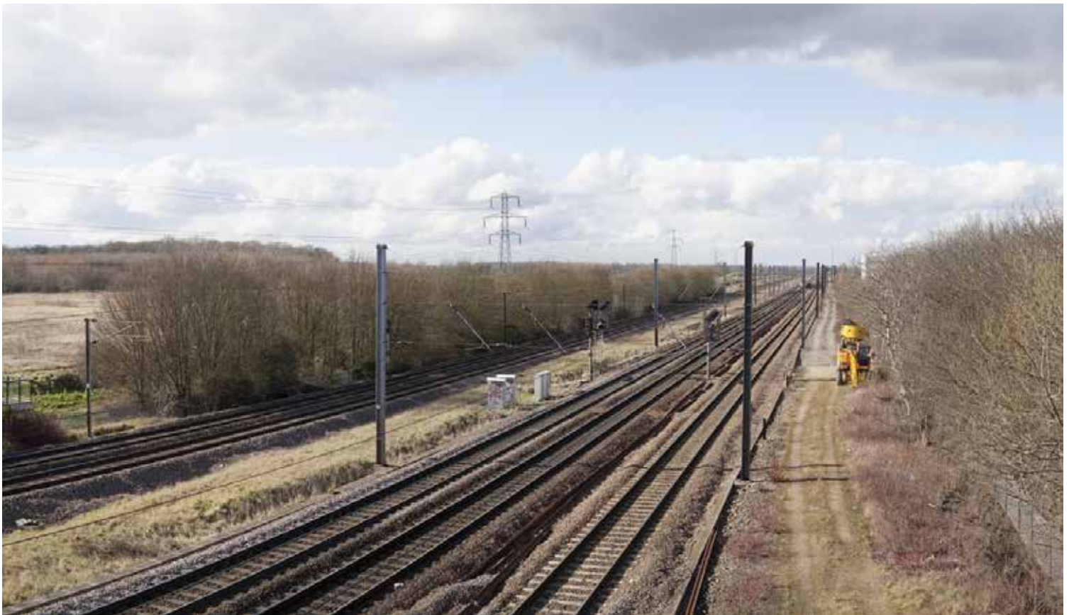
DIVE-UNDER: Network Rail is planning to build a new chord for the East Coast main line near Werrington Junction, Peterborough
