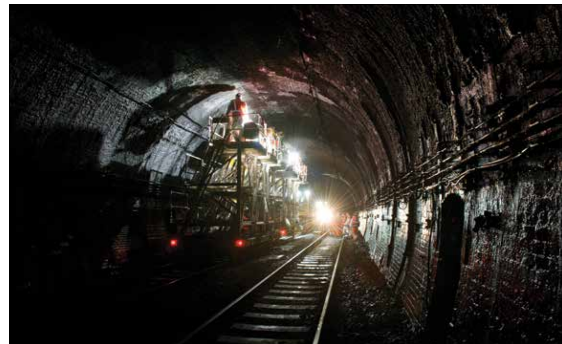
ELECTRIFICATION UPGRADE: Trains between South Wales and London are being diverted until 24 October while electrification work is carried out in the Severn tunnel
