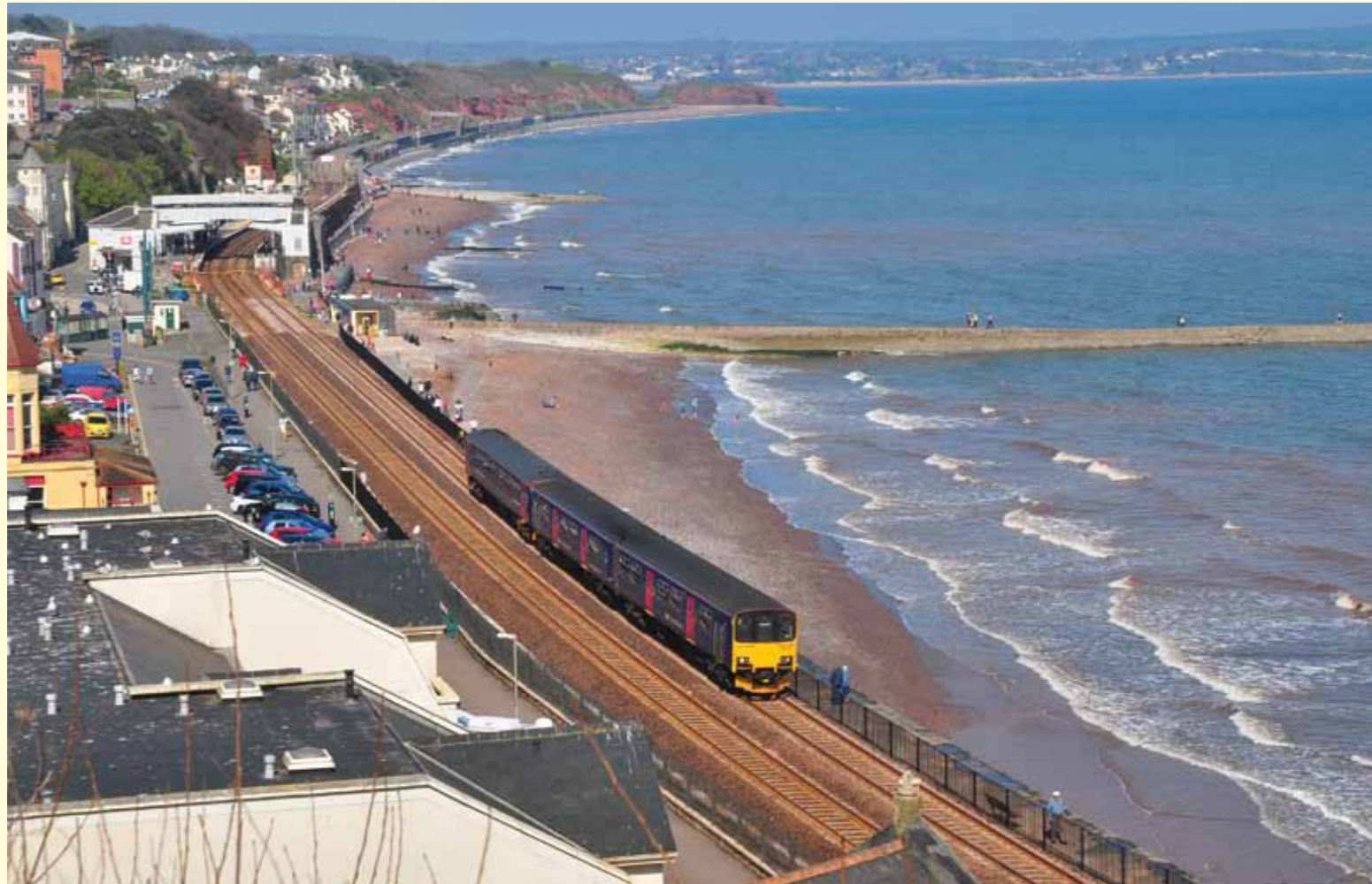
BACK IN ACTION: The sun is shining again as a local train leaves Dawlish, heading west, to areas which were cut off when storms smashed the sea wall and left the track dangling in the air. Repairs took two months
