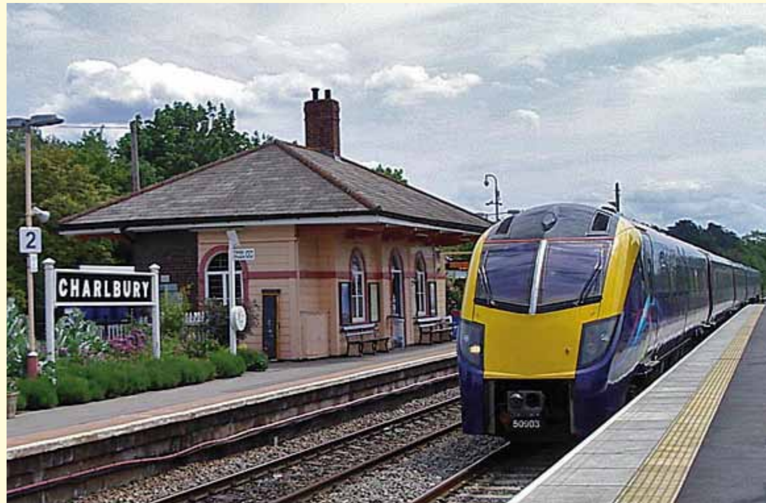
PUTTING BACK THE TRACK: A £70 million scheme restored 21 miles of the Cotswold Line in 2011 to improve reliability. The line was not listed 'for development' in the second Beeching report in 1965 and was reduced to single track in 1971. Here a train for Great Malvern calls at Charlbury's new platform on one of the redoubled sections. In the background is the Brunel station building, while to the left is the memorial garden to former British Rail chairman Sir Peter Parker, who lived nearby and was a regular user of the station
