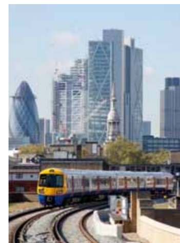
CYBER CITY: The bright new Overground railway services the new silicon industries of Shoreditch and links south London to traditional business in the City
