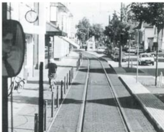
Integrated: Karlsruhe trams goes through streets which have room for cyclists and pedestrians. The trams run through on to the main rail network. Picture: Tony Smale
