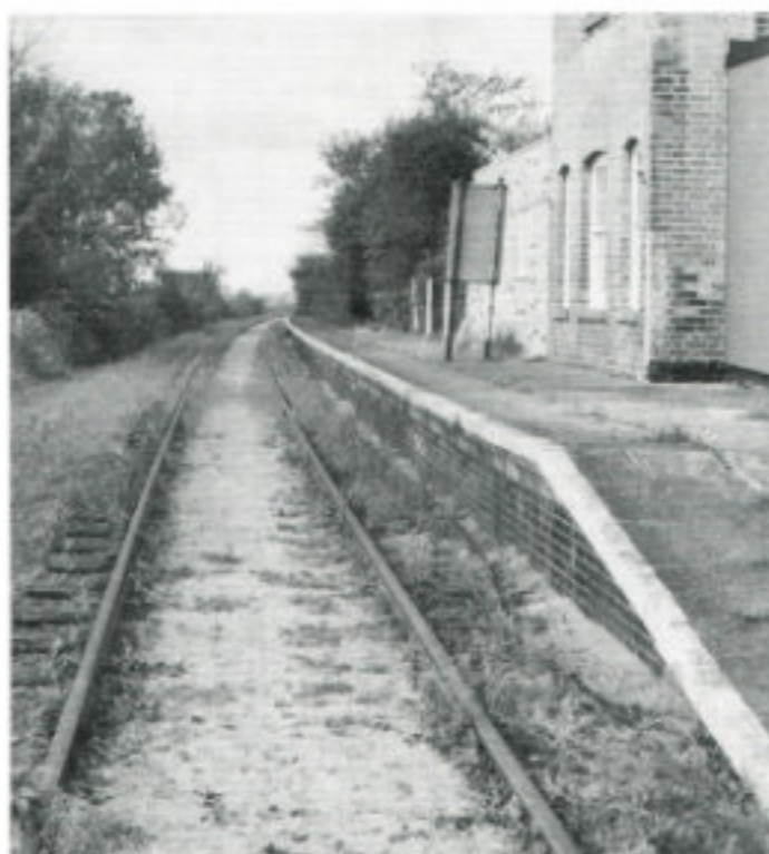
Years of neglect: But the line is still in situ at Oakington station on the Cambridge-St Ives route. Picture: Nick Dibben
