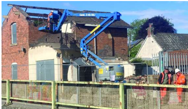
More than just a spade in the ground: Workers on the rebuilding project use an articulated boom lift to dismantle the old station house, reclaiming the bricks for further use and making way for work to start on Pill's new station
