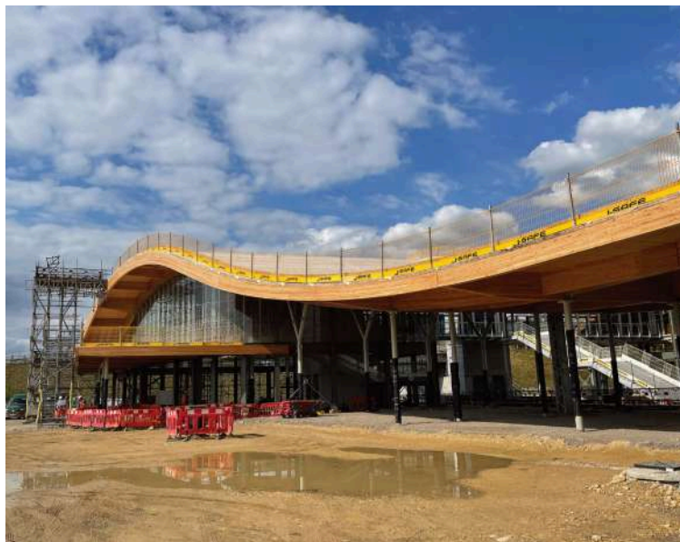
SWEEPING AHEAD: Cambridge South station during construction
