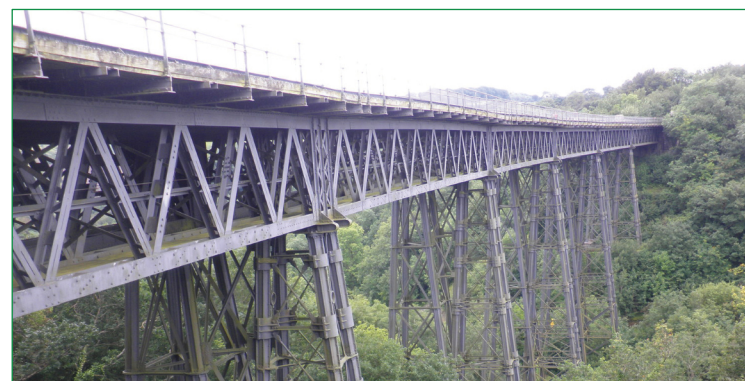
MELDON VIADUCT: A potential alternative rail way to Plymouth
