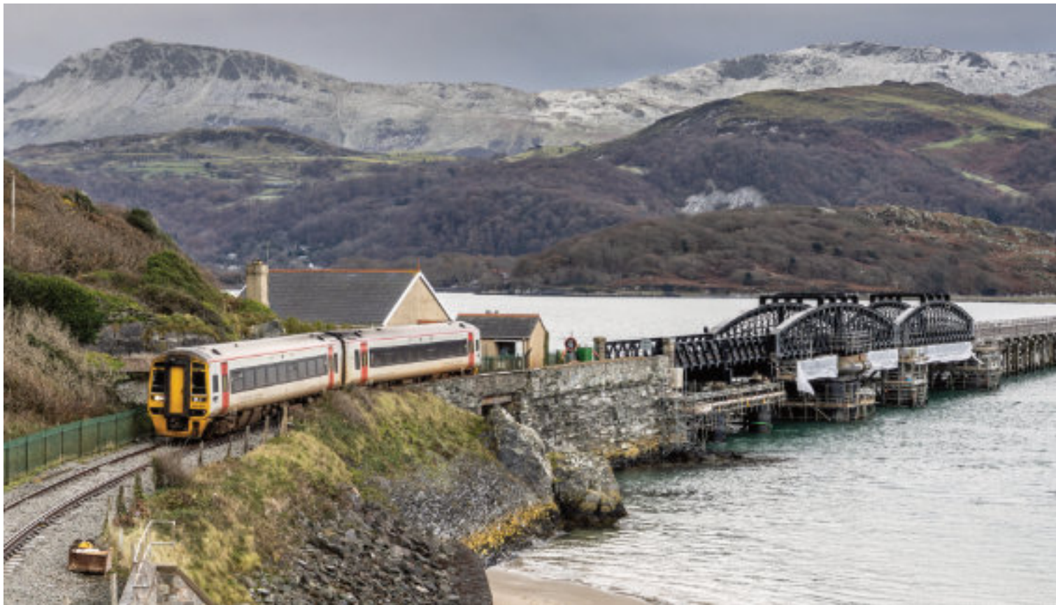
BACK IN ACTION: Pont Abermaw (Barmouth bridge) has been renovated after a major £30 million upgrade. The rail service was suspended for three months in autumn 2023 but resumed in December. Network Rail's picture shows a Machynlleth to Pwllheli train, Afon Mawddach and snow-covered Cadair Idris in the background
