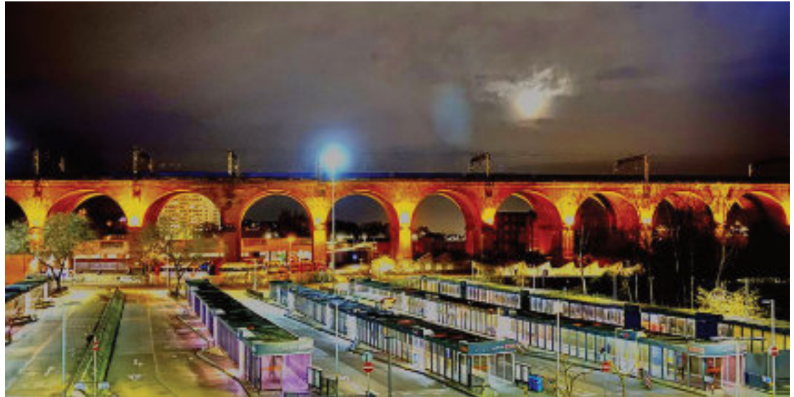
Network Rail is seeking planning permission to repair the 27-span Stockport viaduct over the river Mersey because some of its estimated 11 million bricks are crumbling and other safety measures are needed. Nearby, work is continuing on a new transport interchange to replace the old bus station and to create "improved links to the rail station". The interchange is scheduled to open in March Picture: @every_station
