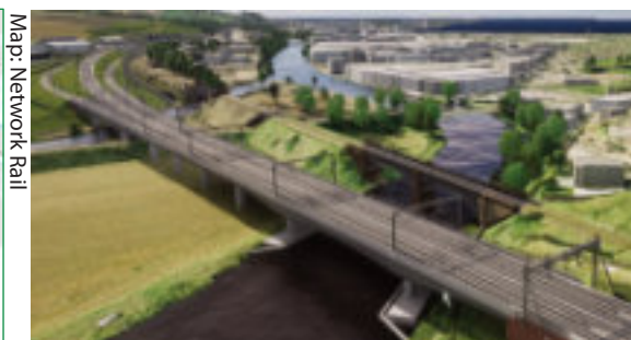
FUTURE: Design for a new four-track viaduct over the river Calder at Ravensthorpe, near Leeds and Wakefield diverge
