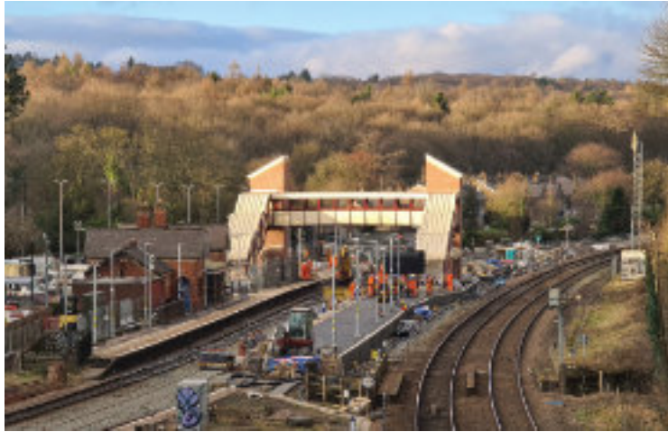
ACCESSIBLE FUTURE: Lifts are installed at Dore & Totley station
