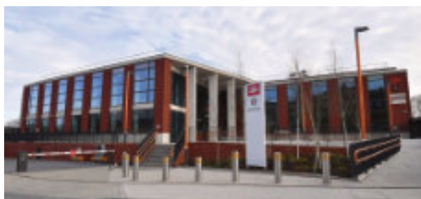
UNIVERSITY STATION Photo West Midlands Rail Executive
