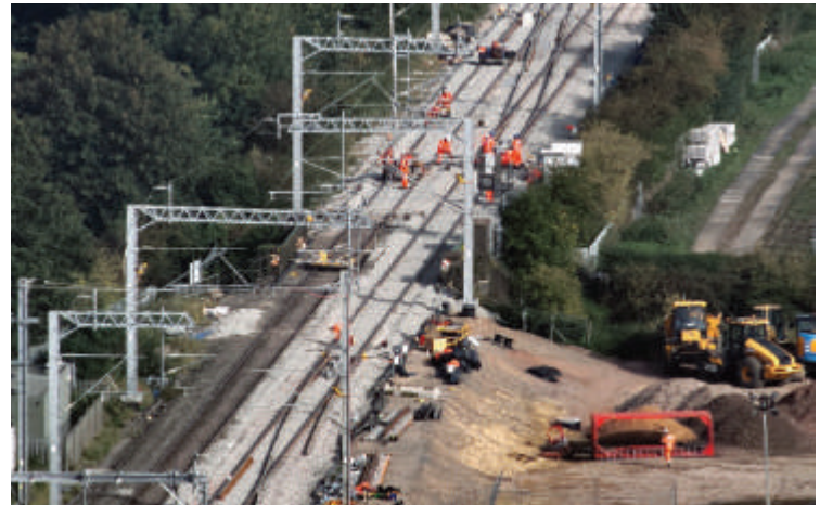
Aerial view of work to connect to main line
