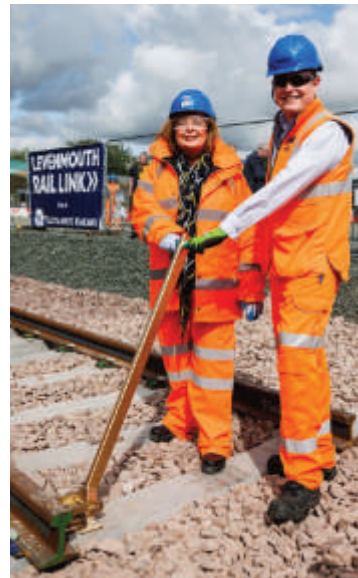
Scottish transport minister Fiona Hyslop installed the final track clip with Alex Hynes, managing director of ScotRail, to mark completion of track laying on the Levenmouth reopening project on 25 August Picture: Network Rail
