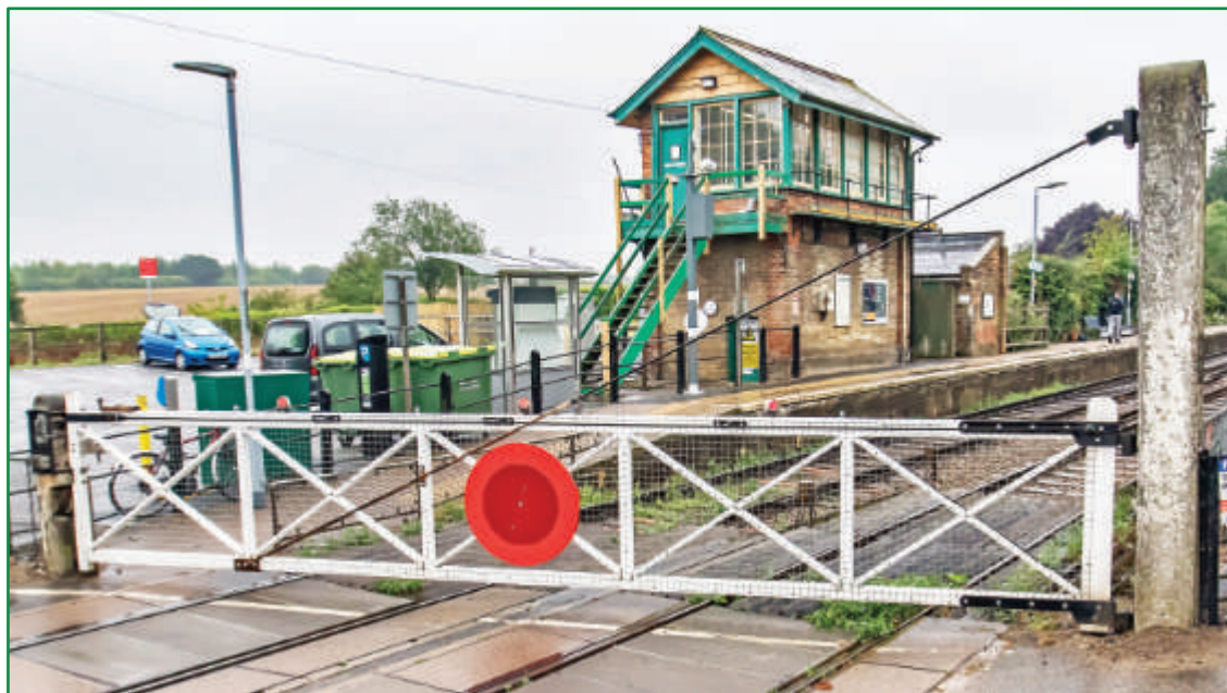
An increasingly unusual sight: Full-width staff-operated crossing gates. Dullingham in August 2021
