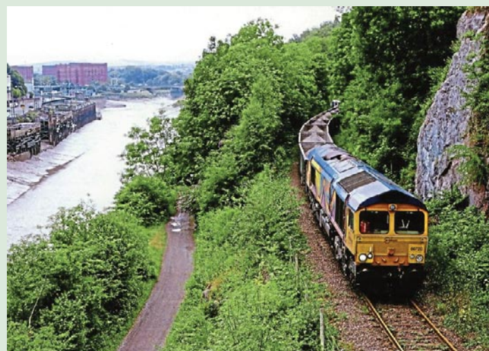
DELAY: Delays have hit the scheme to get passenger trains running through the Avon Gorge to Portishead. At present, the line is used only by freight trains to Portbury Docks
