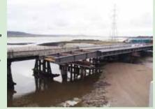
new double track, to provide extra capacity and flexibility for passenger services on the main line to and from West Wales. Gowerton's eastbound platform will also be reopened. Sections of the existing bridge which is a timber structure, will be preserved in the new structure.
