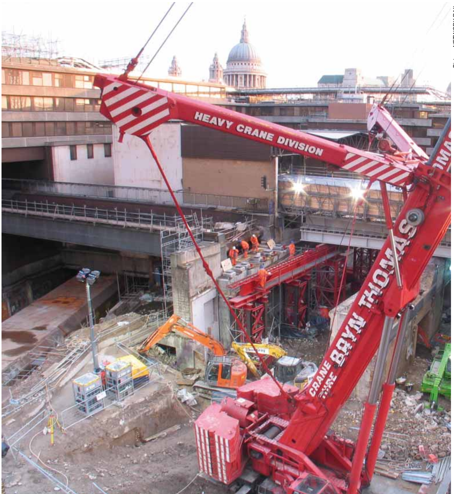
Picture: NETWORK RAIL
