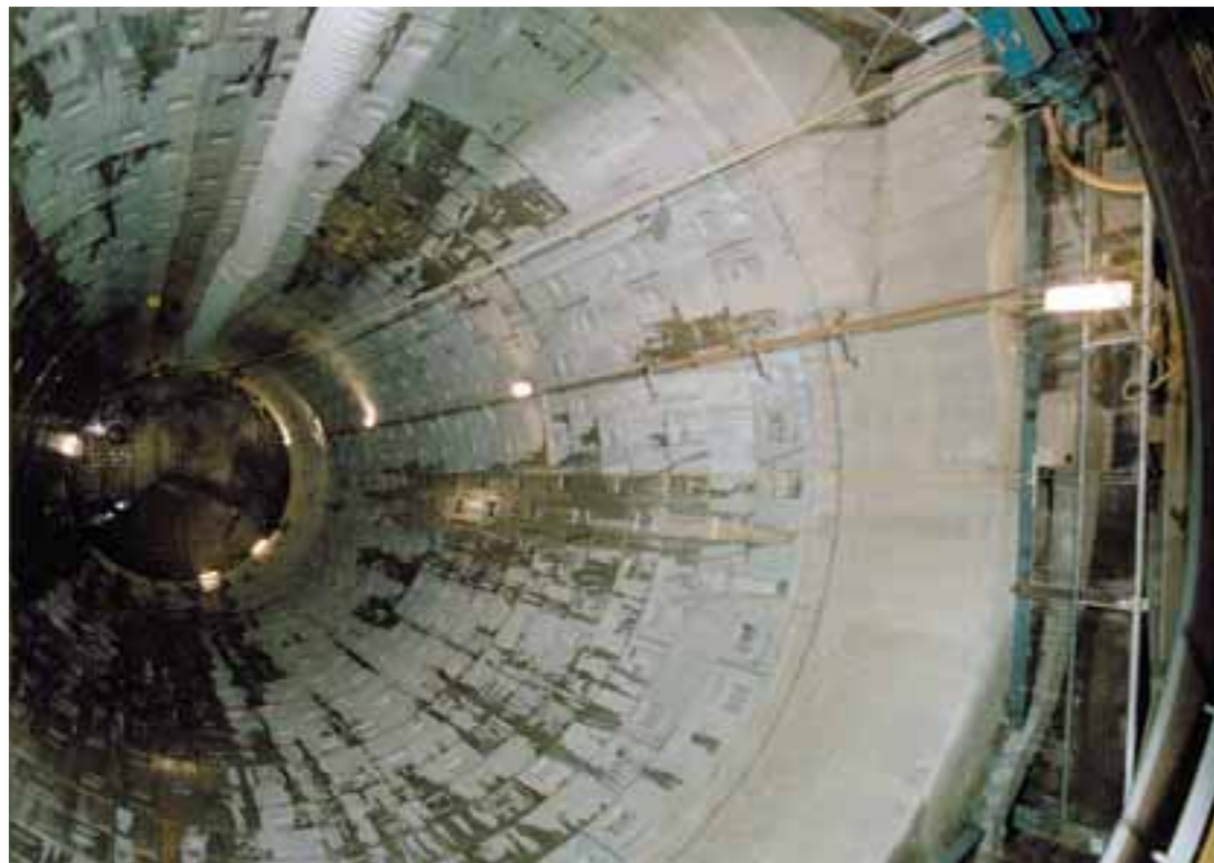
LONDON CROSSRAIL: A 34-metre ventilation shaft has been built at Moorhouse in London. A station will be built at the foot of the shaft. But the go-ahead for the whole scheme was still awaited in September. More info: www.crossrail.co.uk
