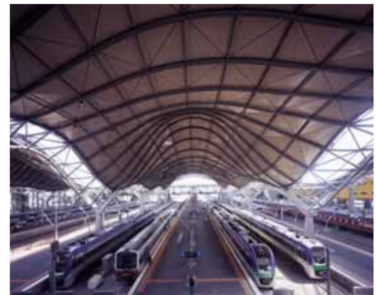
2007: Melbourne's new Southern Cross station designed by British architect Nicholas Grimshaw Picture: Shannon McGrath
