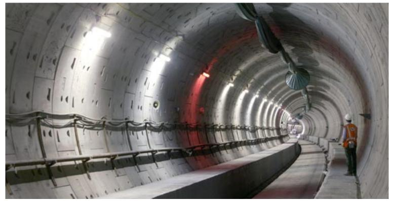
Concrete track beds and walkways were being laid this summer in the second stage of Britain's first high-speed line. The work was under way between Stratford and Manor Park in East London and Dagenham, Essex, prior to track-laying, signalling and electrification.
