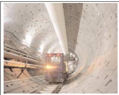
This picture shows a narrow guage works train fitting out the new Channel Tunnel rail link tunnel under the River Thames.
