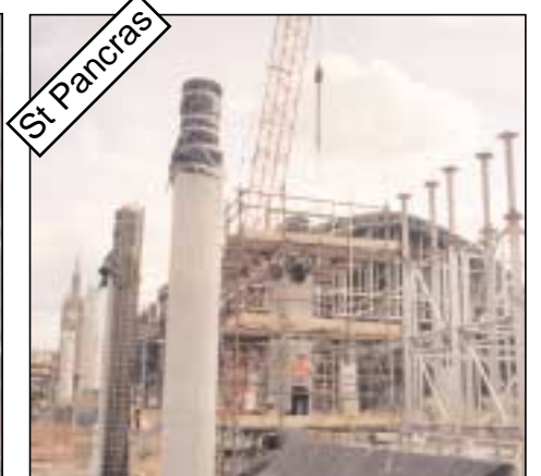
Work starts on the extension to St Pancras station in London
