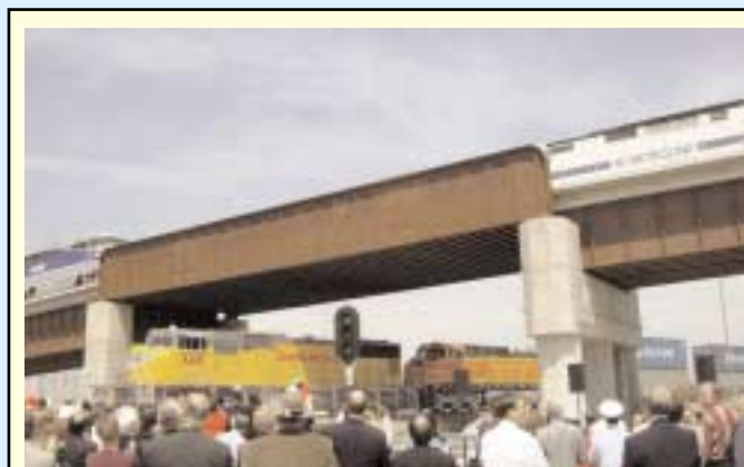
The Redondo Junction railroad bridge provides a faster route for Amtrak and Metrolink trains in and out of Los Angeles Union Station. This grade separation eliminates a conflict between freight, passenger and motorists. The bridge was completed in August and commuters on the Amtrak and Metrolink enjoy a faster and efficient ride in and out of Union Station without holding up freight trains.
