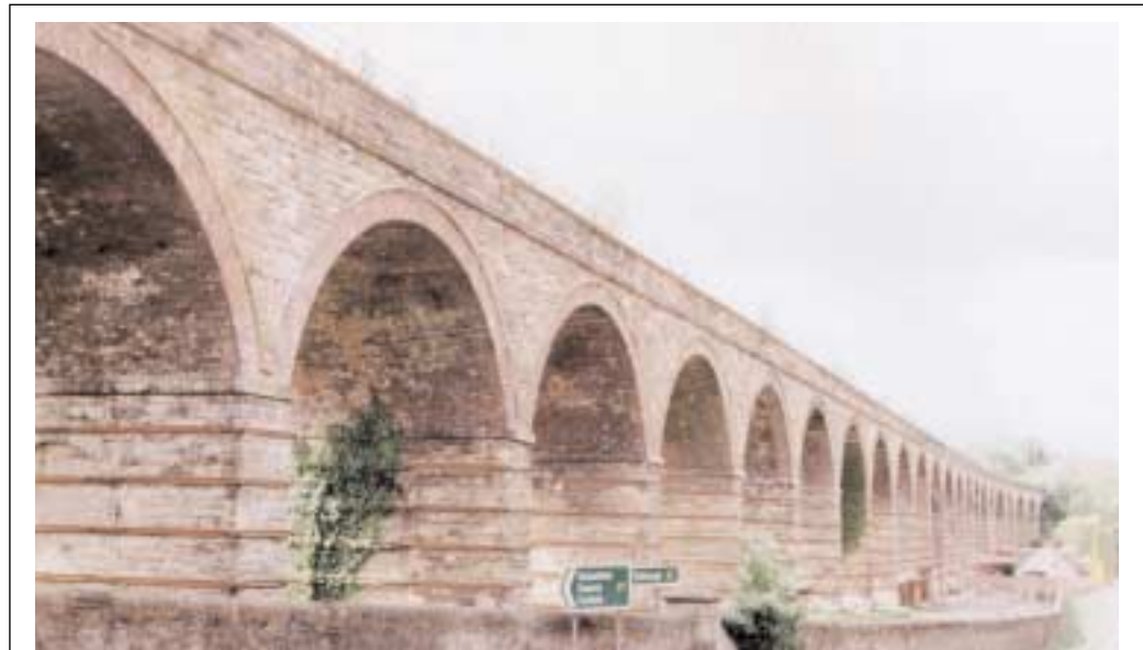
This beautiful viaduct at Newbattle, out of use for 30 years, may soon see trains again following a report which says that at least part of the Waverley route could be reopened to serve the Scottish Borders. The viaduct, near Dalkeith, has survived but many other parts of the line have been blocked by roads or building of other sorts. If protection had been effective the whole line could have reopened. Report: Back page Picture: Scott Wilson
