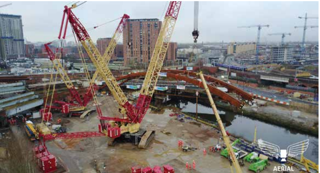
MANCHESTER: A crucial step in improving northern England's rail network was achieved in February when this structure for the Ordsall Curve was lifted into place. It will link Manchester's main stations. Network Rail said it is also Britain's first asymmetrical network arch railway bridge
