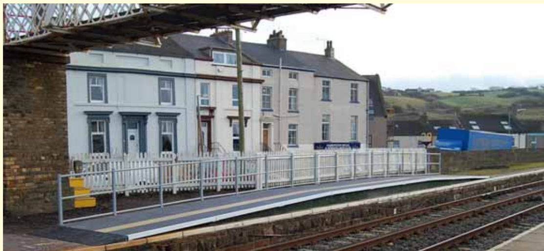
CLOSING THE GAP: The Harrington hump improved access and saved more than £200,000
