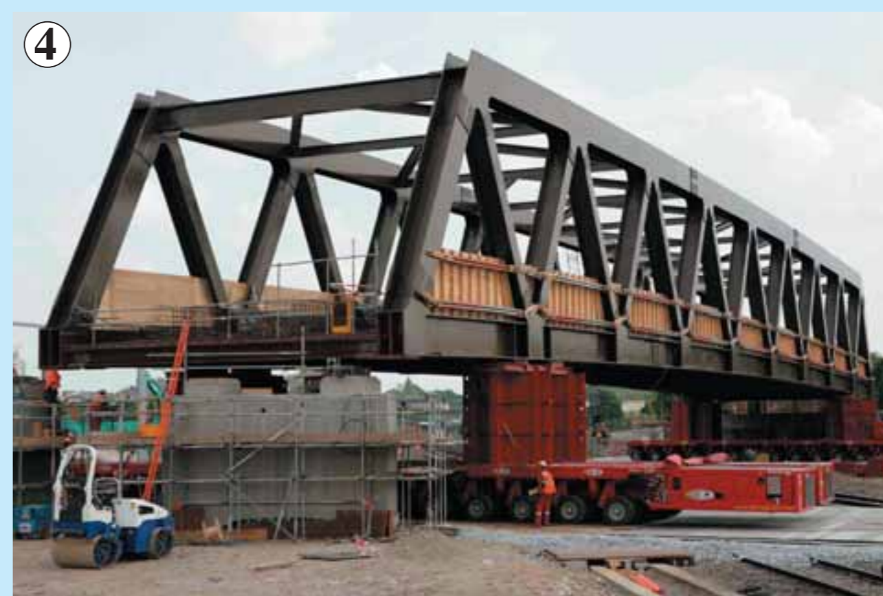
SHOREDITCH HIGH STREET: This 350-tonne bridge was lifted into place with Britain's biggest mobile crane in March 2008
