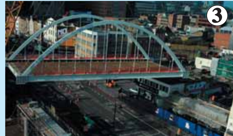
SHOREDITCH HIGH STREET: This 350-tonne bridge was lifted into place with Britain's biggest mobile crane in March 2008
