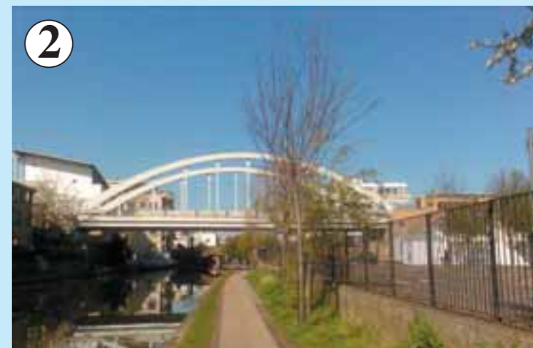
HAGGERSTON: The first bow-string bridge for the East London line extension was built over the Regent's Canal in 2007
