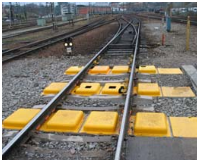
TRACK WATCH: The VIEW TM Technology checks for worn components on trains
