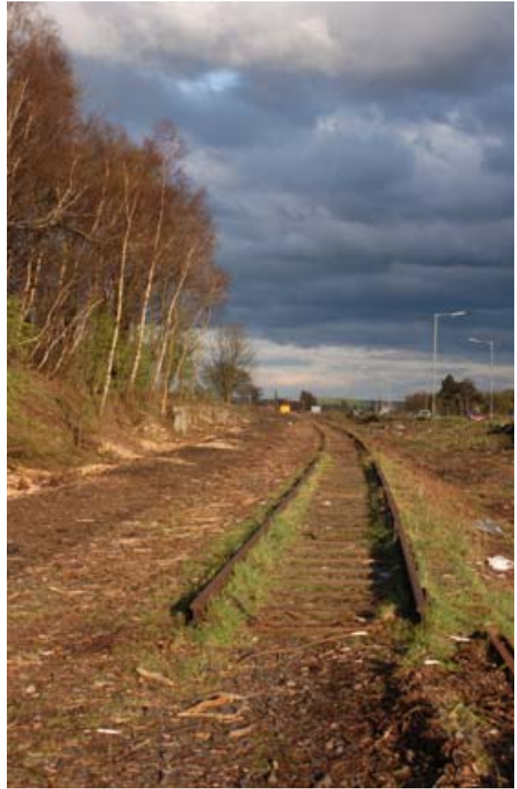
Stop the rot: This was the line looking towards Dunfermline in April. Now work has started on reopening Picture: Railphotolibrary.com
