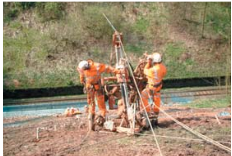
Chorley cutting, with abseilers at work
